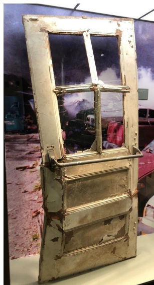
A metal door from the building after the blast.
