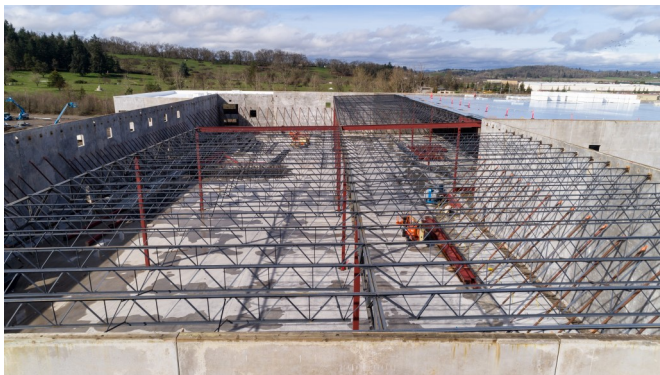
Yogi Tea Roof Trusses
