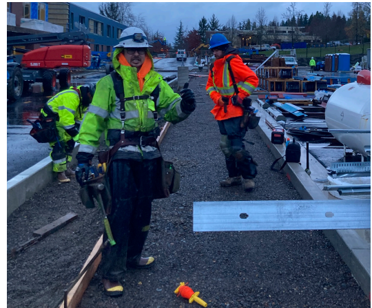
Subcontractors ready for the rain at Camas Ridge!
