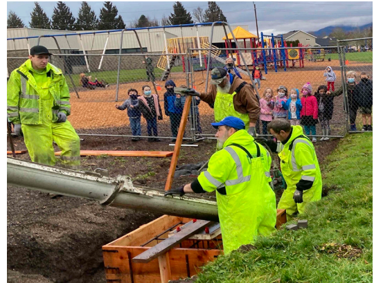
Our team in their rain gear pouring concrete at Gilham
